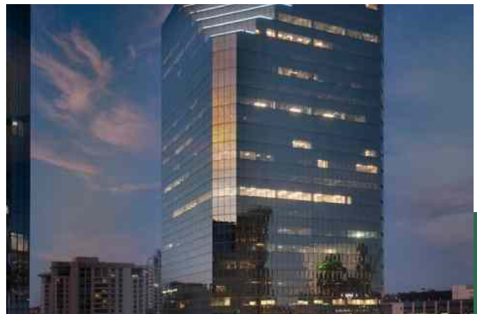
Photo Copyright © Baker Electric
